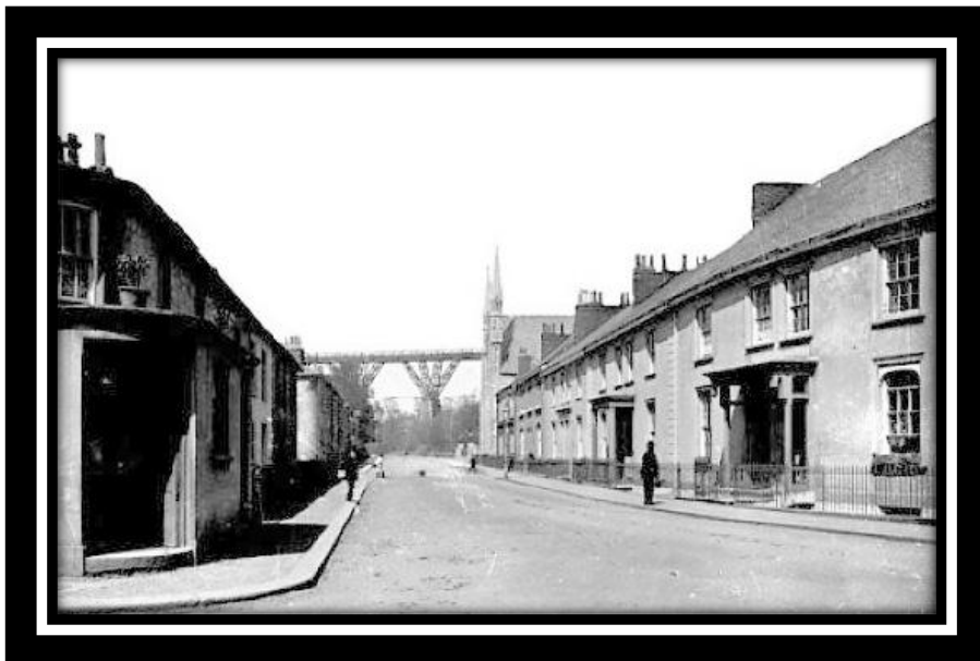
Ferristown Inn on the left (Photo - courtesy of Paul Caruana)
