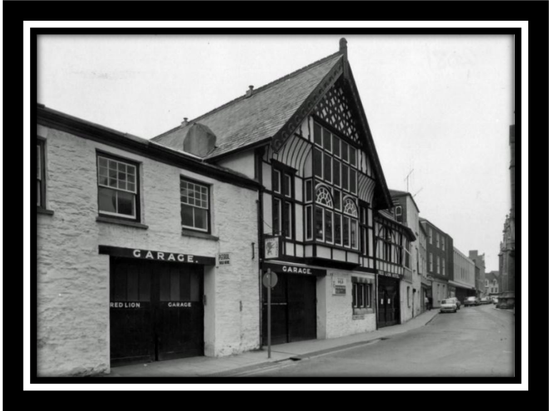
The rear elevation in St Mary's Street
