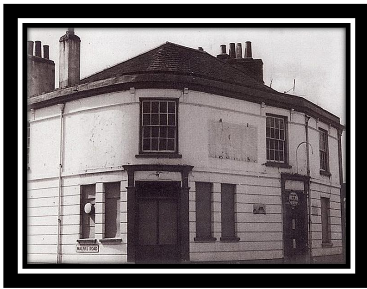
The Admiral Boscawen ready for demolition
